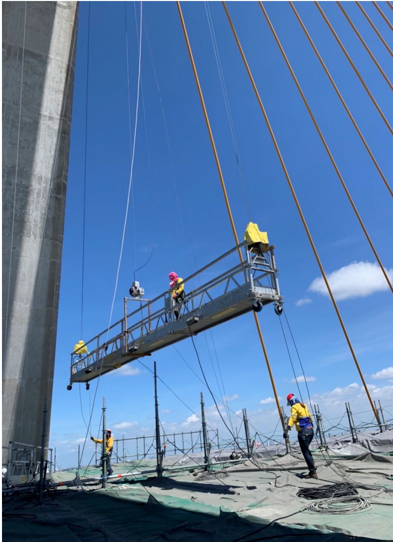
Installation and Dismantling
